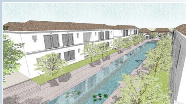
Aerial view of the hotel guest block
