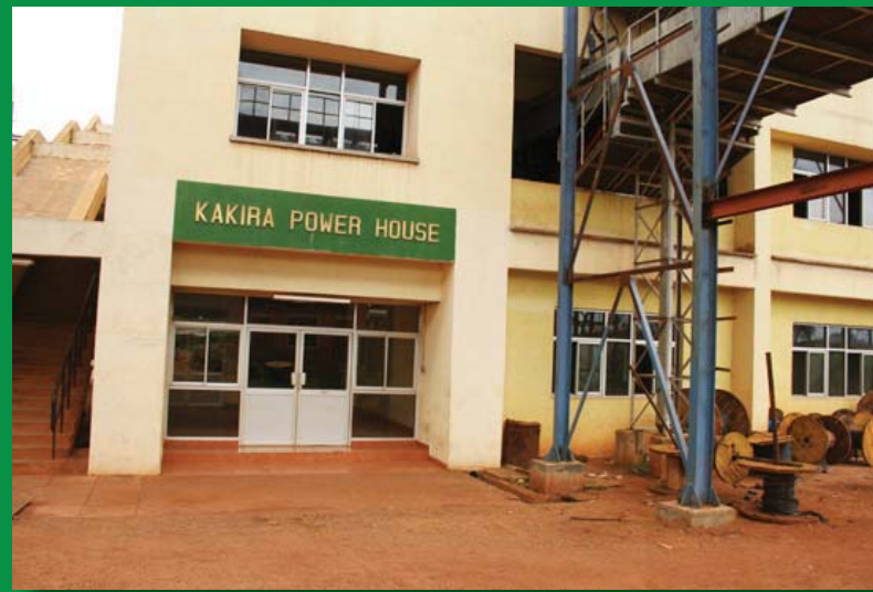
Entrance to the Kakira Power House
