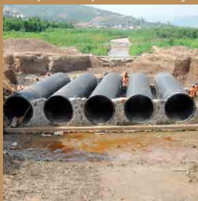
A marshy area in Kabuye before and after bridge construction
