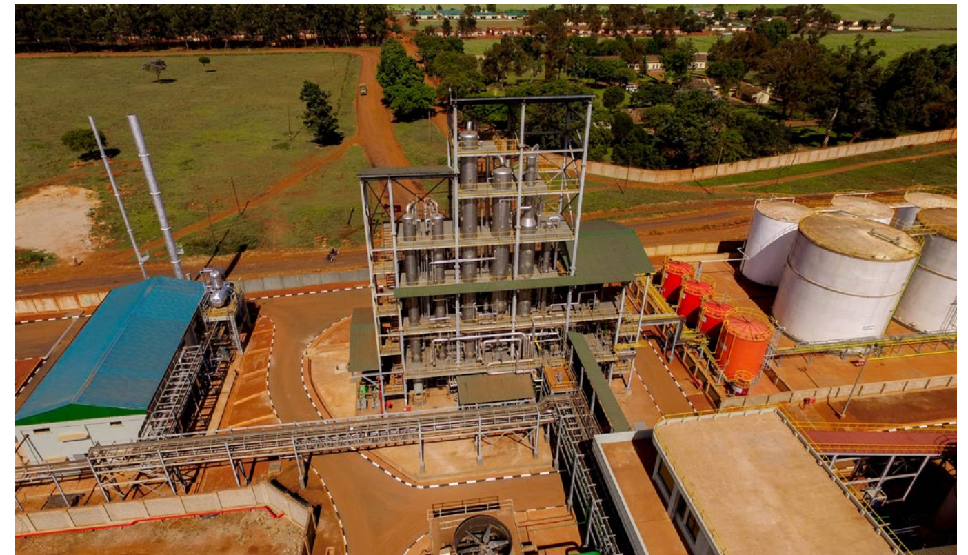
An aerial view of the distilling facility at Kakira Sugar Limited
